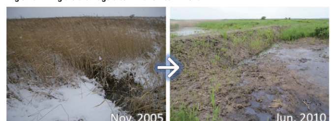
Fig.5 Damming the drainage ditch with embankment
