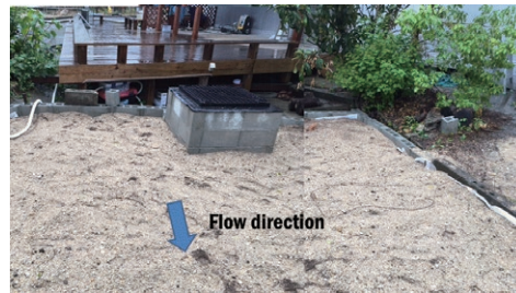
Photo2 Rain garden located downstream of the rain water storage tank
