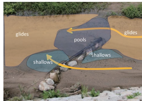
Fig.15 Diversification of water flow by log structure (downstream direction)
